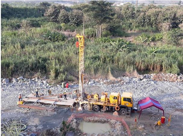
Water well drilling with a PRAKLA RB 40 rig in Ghana
